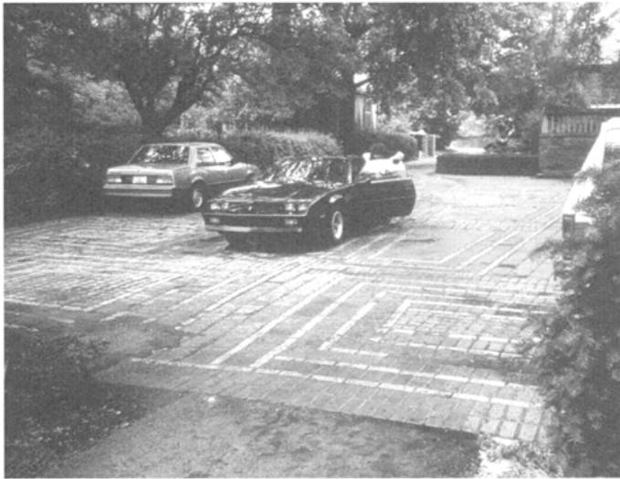
Fig. 13. Unit pavers at Cranbrook.
